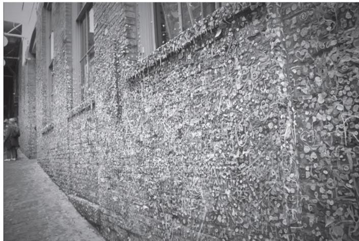
Figure 1: Side view of the wall before it was cleaned.
